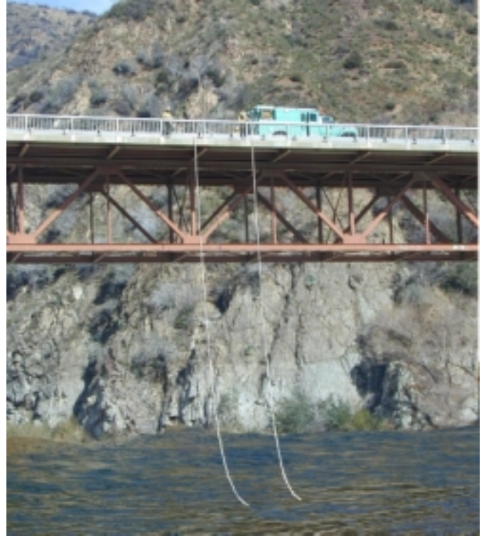
Figure 7—Ejector operation from a bridge.
